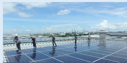
Maintenance (module cleaning)
